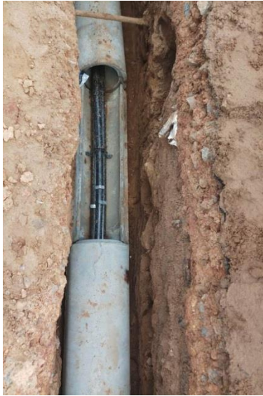
UG Cabling for 33kV & 11kV
