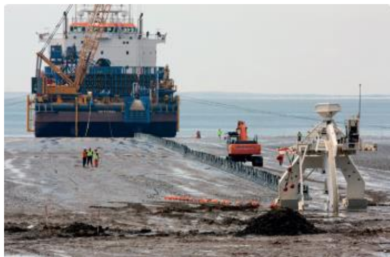
Figure 33: Cable barge and plough making landfall [31]
