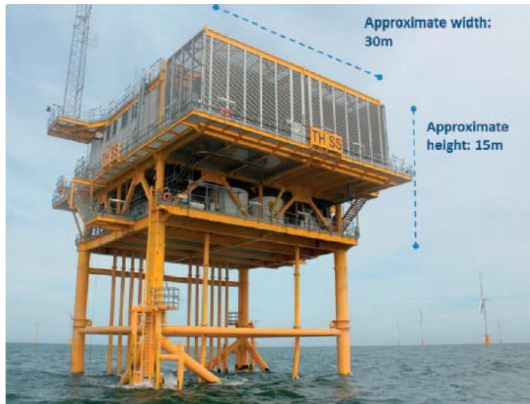
Figure 29: An example of an offshore HVAC Substation [31]
