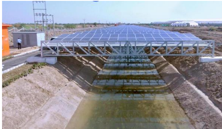
Fig 3-12: solar project on Narmada branch canal network (1 MW)
