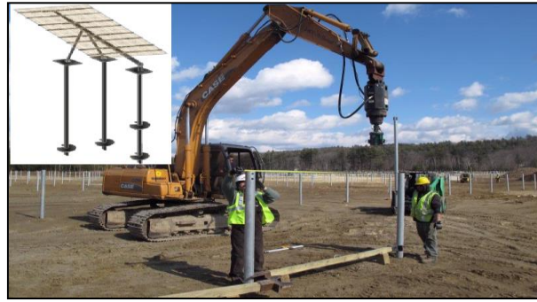
Fig. 6-4 Helical Foundation – Crawler mounted driller
