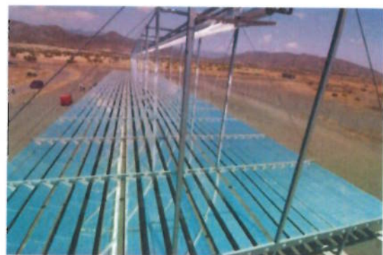
Fig A10: which will be the largest Fresnel power plant with 30 MW electric power (source: Novatec Solar)
