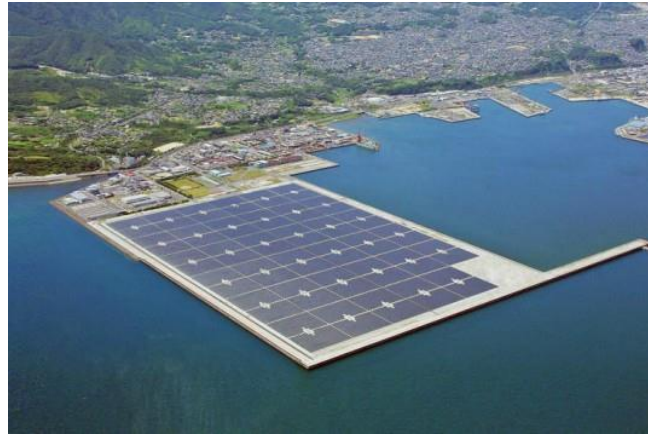
Fig 3-8: Kagoshima Nanatsujima (Japan) Mega Off shore Solar Power Plant (70MW)
