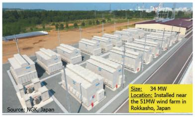
Figure 7-10: 34 MW NaS Battery Storage in Japan
